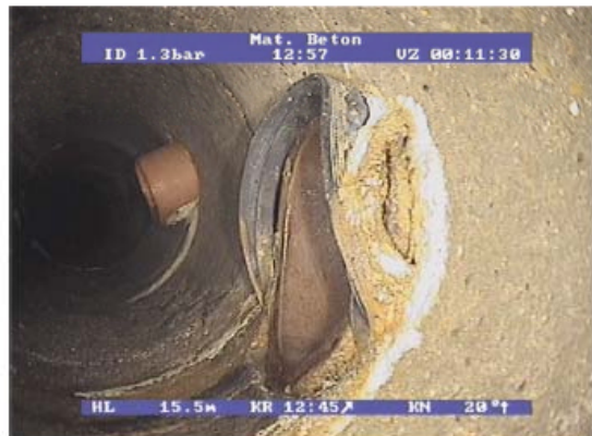
defekte Anschlüsse
